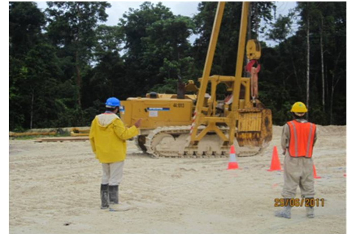
Pipe layer (sideboom) training
