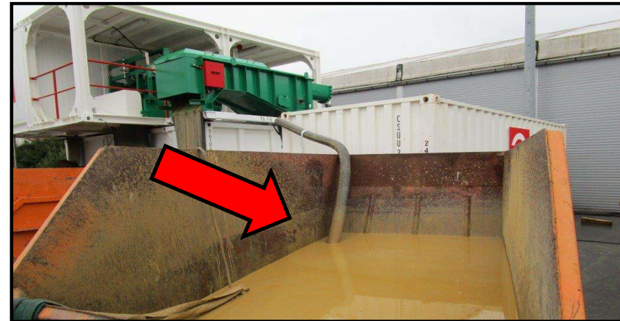
Untreated drilling fluid is pumped upwards.
