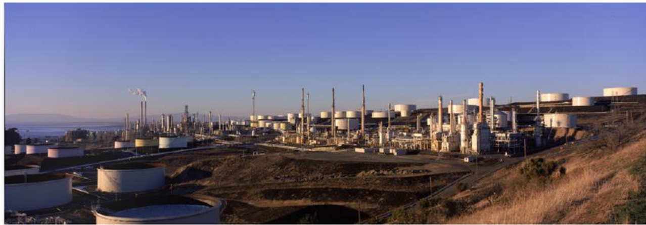
Trans Anatolian Natural Gas Pipeline Project
