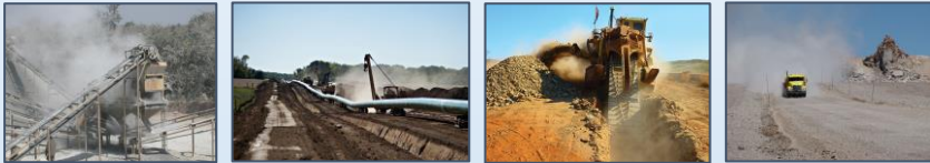
In pipeline construction, major sources of SiO 2 are trenching, crushing and road construction.
