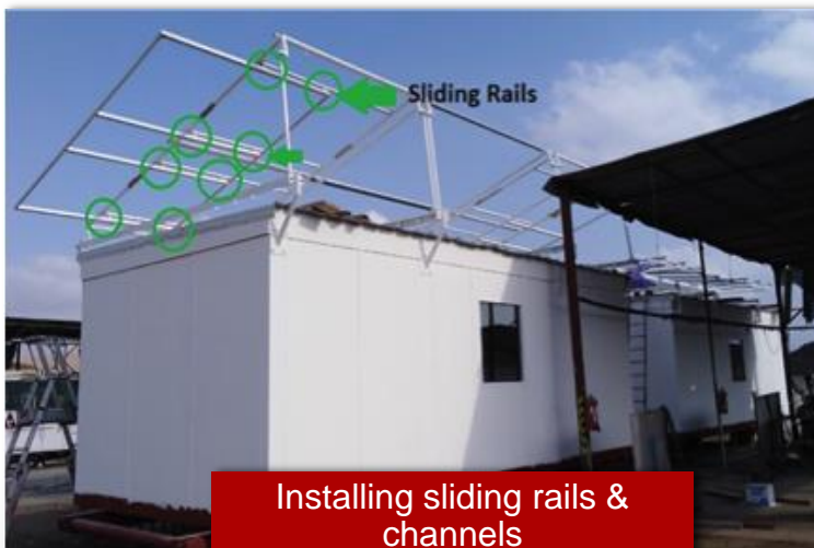
Assembling PV frames & windows
