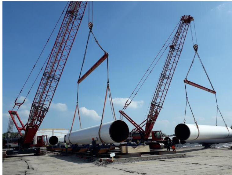
Figure 4-6 Pipe handling on the double jointing yard
