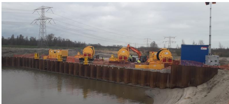
Figure 4-44 Mainland winch set-up (phase 2)
