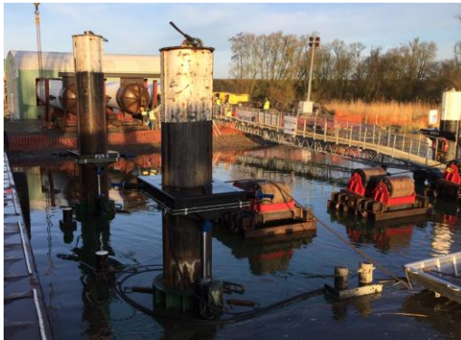
Figure 4-24 Jack-up pontoon with rollers
