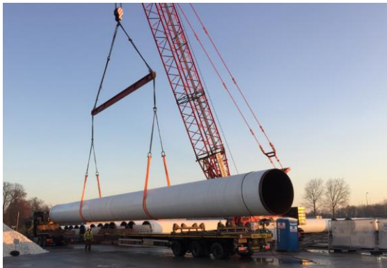
Figure 4-9 Pipe loading storage area
