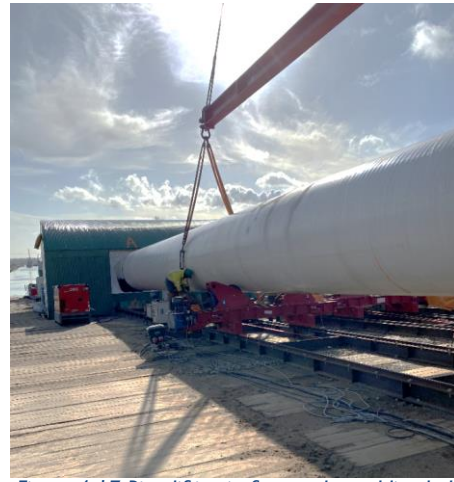
Figure 4-17 Pipe lifting in front a the welding hall
