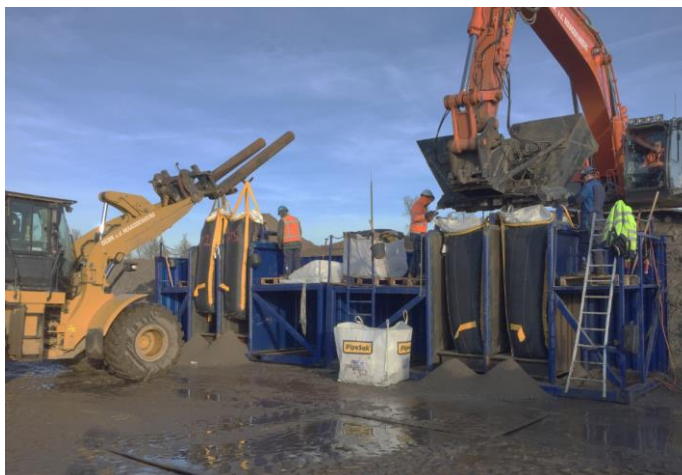
Figure 4-32 PipeSak filling set-up
