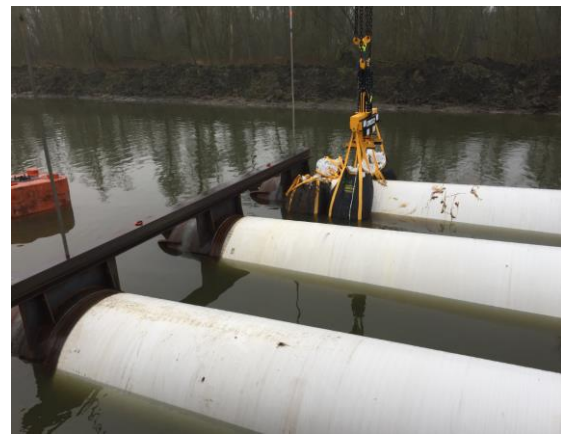
Figure 4-40 PipeSak installation with crane vessel (2)
