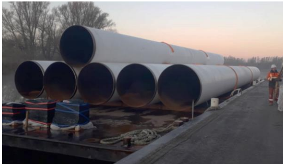
Figure 4-11 Unloading pipe pontoon at the 'Kerksloot'
