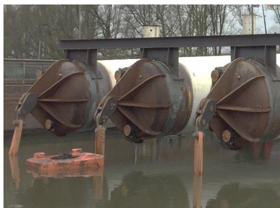
Figure 4-6 Pull-heads with welded spacer profile on top
