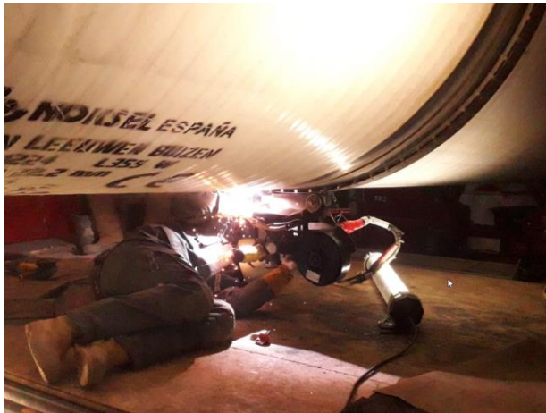
Figure 4-19 FCAW with CRC bug
