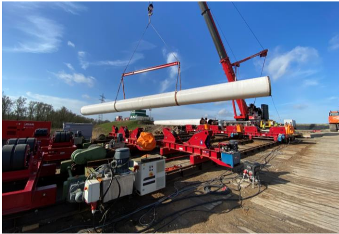
Figure 4-16 Installation of a double-joint on the first hydraulic-driven roller section
