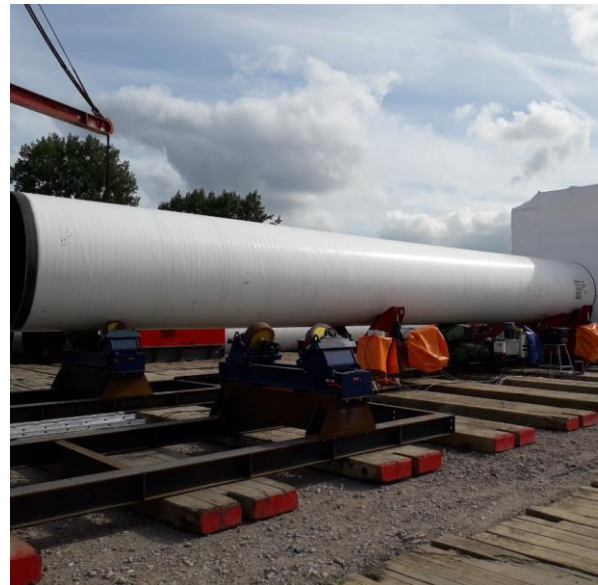
Figure 4-4 Rails & rollers set-up, welding tent
