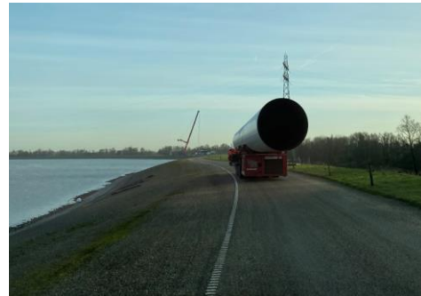
Figure 4-14 SPMT driving on dike
