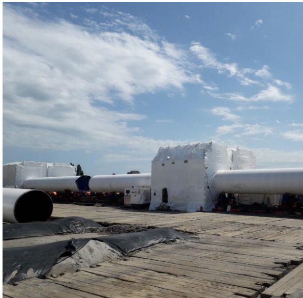
Figure 4-3 Double-joints prefab location in Dordrecht
