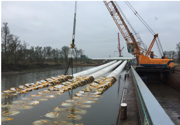
Figure 4-39 long chain installation with crane vessel
