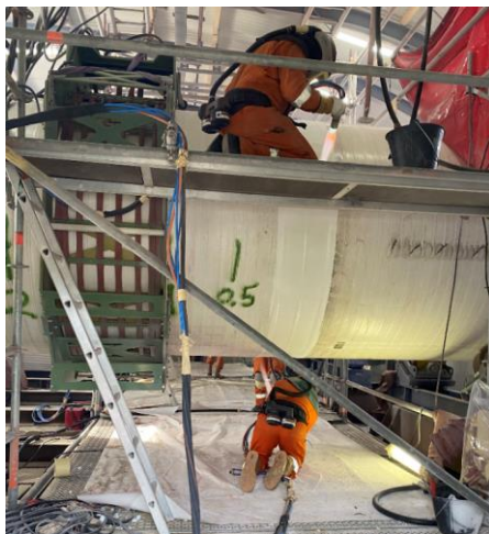
Figure 4-21 Coating with PP-flamespray
