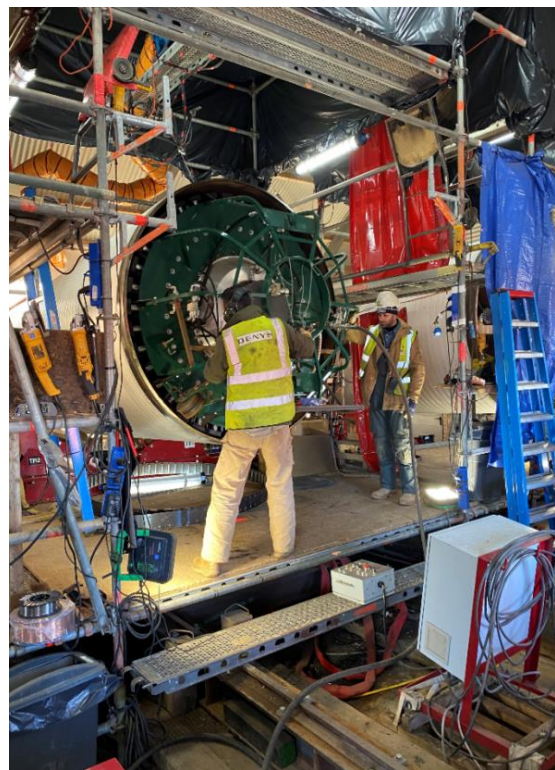
or more specifically TOFD (Time-Of-Flight-Diffraction). Figure 4-18 Pipe fitting with internal clamp
