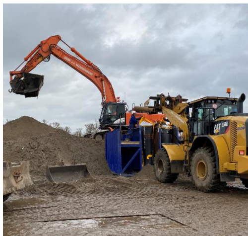
Figure 4-33 PipeSak filling set-up (2)
