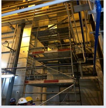
Brief Description During the dismantling of the scaffolding inside the compressor building, a piece of scaffold toebord was dropped from 2.5 meters height and hit the face of the worker standing for dismantling.
