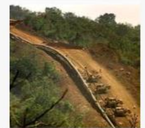
Panvel Dabhol Pipeline Project–Gail Ltd - Maharashtra
