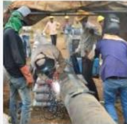
Thumbli Water Pipeline– Cairn Energy India – Rajasthan
