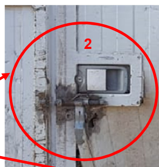
Detail of the original lock (1) and of the modifications made outside (2) and inside (3) the cabin
