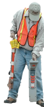
CAT Scanning for UG Utilities
