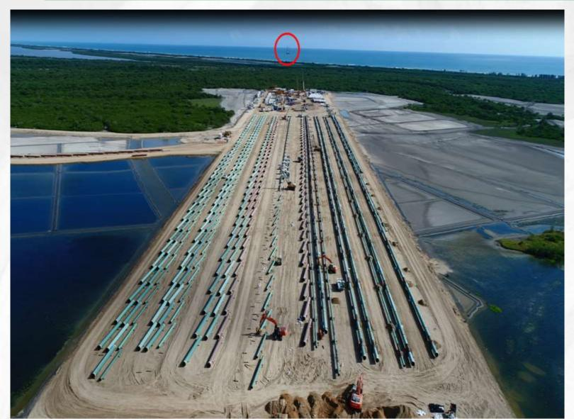
Terratest/Eurohinca microtunnel by pipe-jacking method, 2.2km in length, 3.2m OD, 2.6m ID
