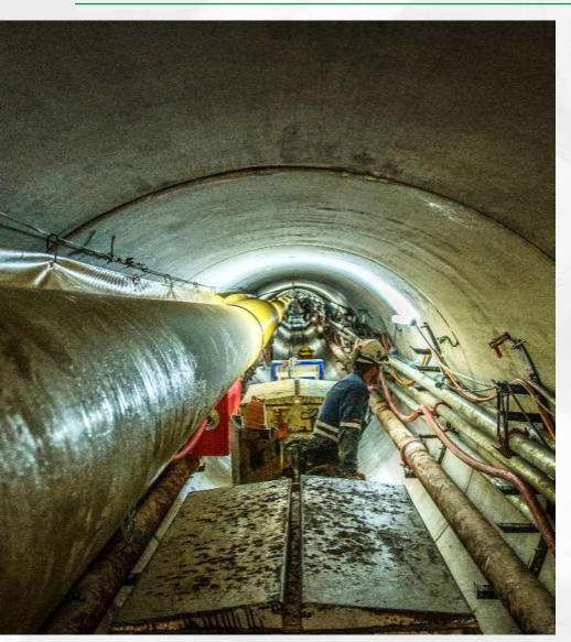
Rail system installed for miniature locomotive for movement of people and materials
