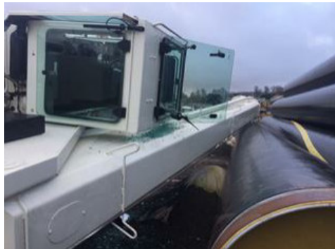
Final position of the crane with the boom on the pipe
