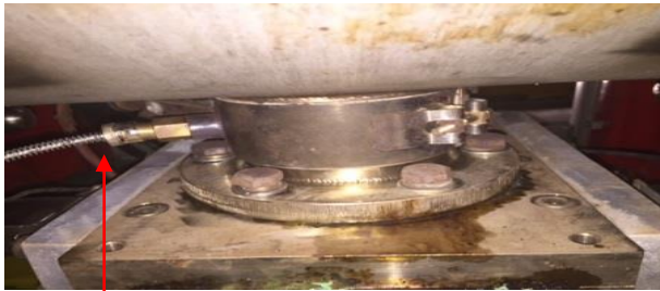
Thermocouple
