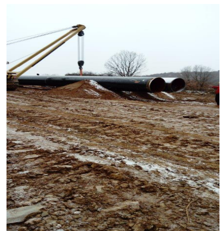
The layout at the moment the pipe slipped
