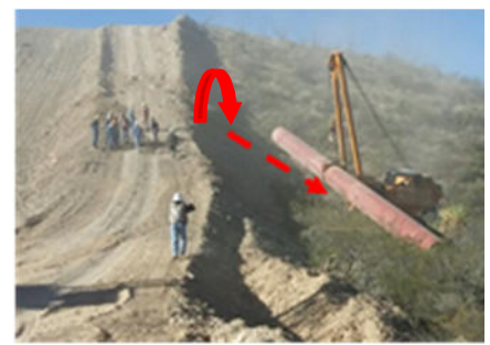
Point where the sideboom starts to rollover
