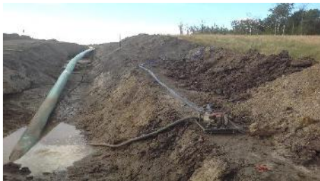
Excavation that was being dewatered. Water was being pumped up hill
