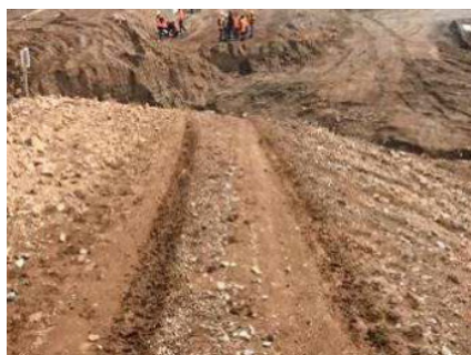
Incident Location: view of the driver
