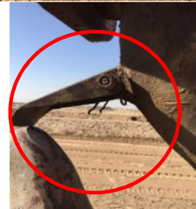
Above the pipe fell down and the damaged hook safety latch.
