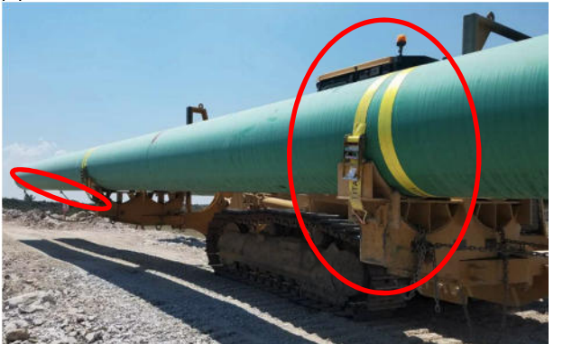
Above: pipe fell off and failure of chain; Below: use of proper ratchet slings for secured the pipes.
