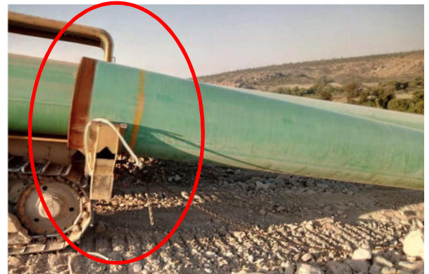
Above: pipe fell off and failure of chain; Below: use of proper ratchet slings for secured the pipes.
