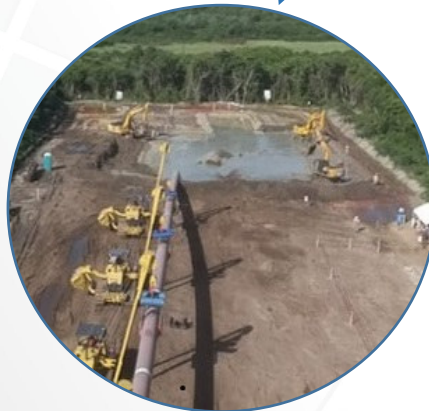
(4 conventional & 2 including NPS 62" casing installation)
