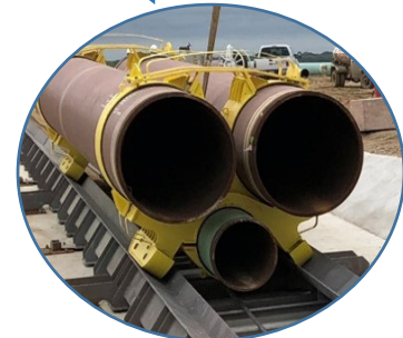
(2 x 42" and 1 x 24" pipe strings stripped together)
