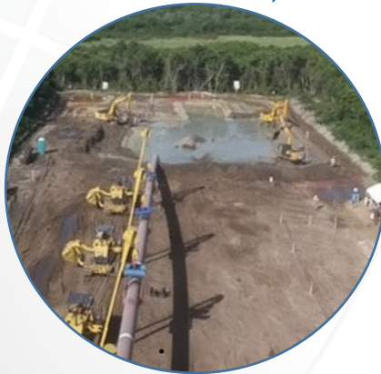
1 NPS 42" conventional HDD crossing
