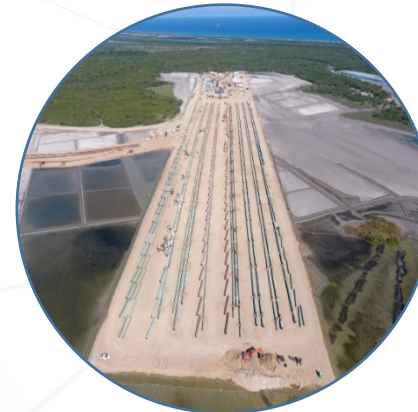
Landfall Platform 800 m x 130 m in a swampy area
