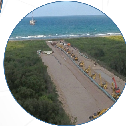
Landfall Platform 885 m X 50 m in a swampy area
