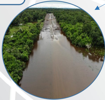
Ground Conditions (Tamiahua Lagoon)
