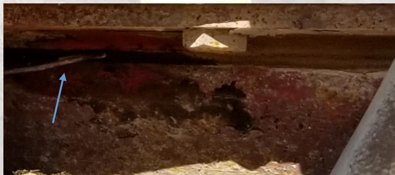
Picture 5: Vertical separation of top and bottom portions of turntable when lifted. Wire in between gap is approximately 3 millimeter
