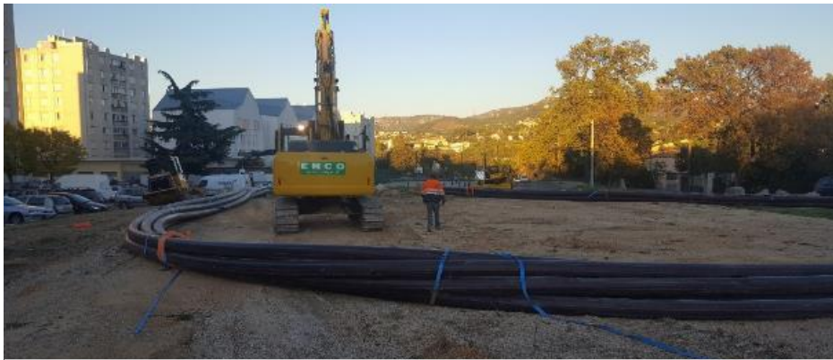
Preparation of pipeline bundle on Pipe side
