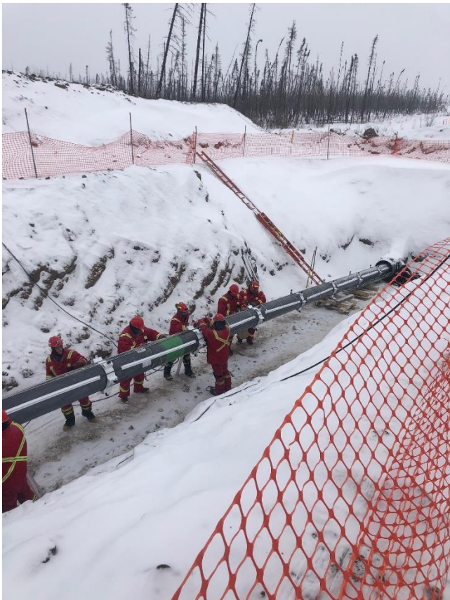
Winter Pullback, attaching spacers
