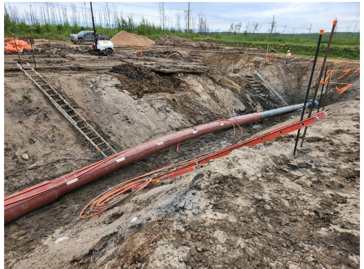
Final position, Overbend attached
