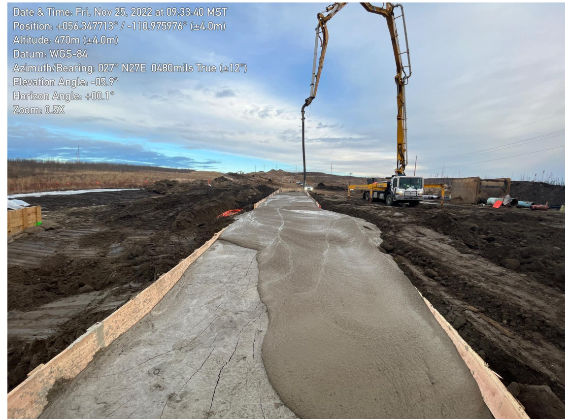
HDD Exit with “fillcrete” overburden
