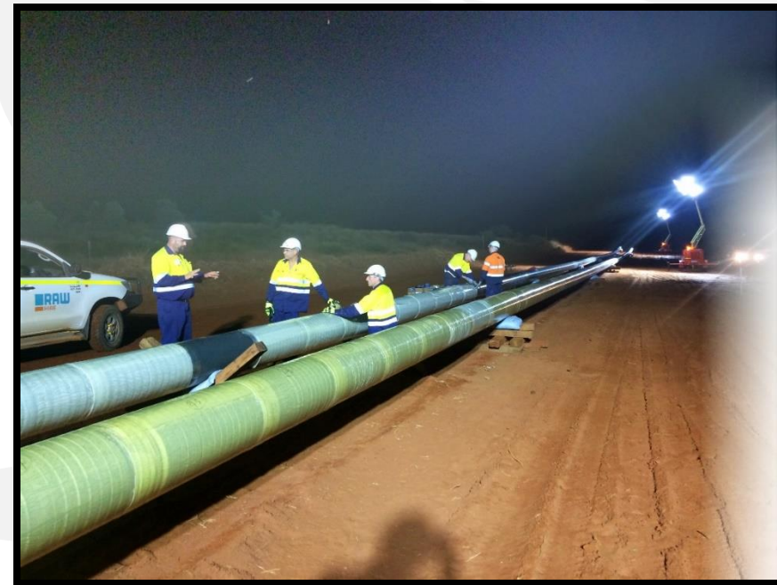
Example of Overnight application to avoid too fast curing
