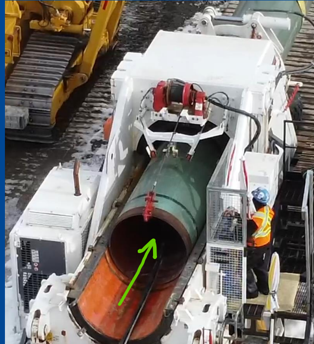
Bending completed and pipe is pulled out
