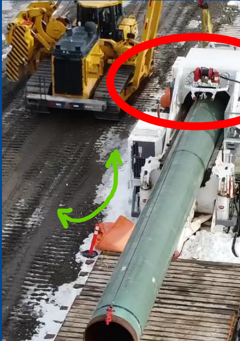
Standard bending operation ongoing
