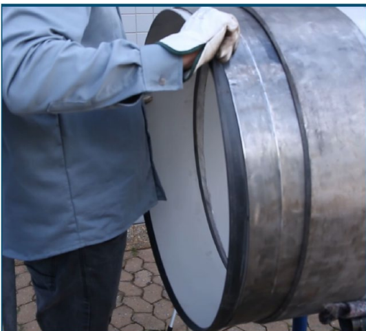
2 nd Bore Seal Installation
