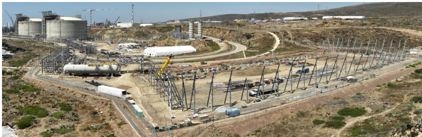
Ground Flare & Refrigerant Storage
