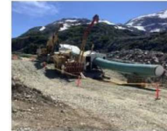
Photo shows pipelayer and Shack setup on pipe section.
