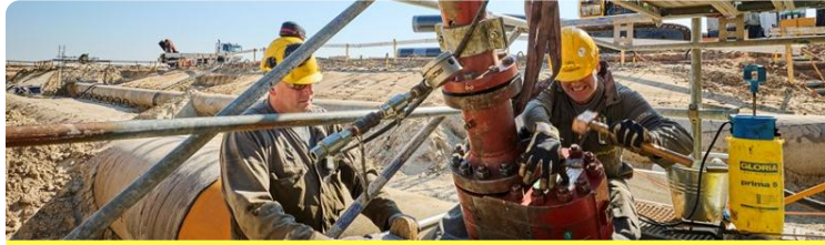
Business line Hydrogen transmission
