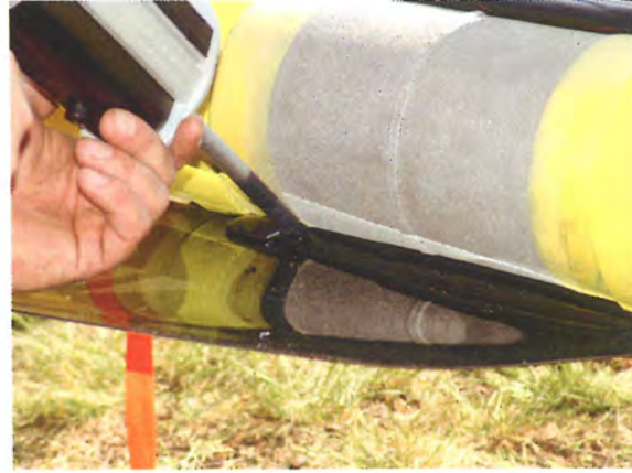
Fig. 3: Application of DENSOLID HDD (casing system). a) closing of casing by means of a bracing bar, b) filling of annular gap from two chamber cartridge, c) overlap of casing ends, d) removal of spacer after removal of casing, e) finished and bevelled joint coating, f) joint coating passing pipe supports.
