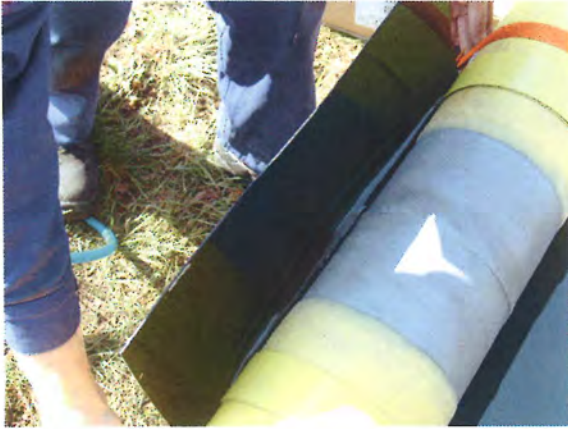
Fig. 3: Application of DENSOLID HDD (casing system). a) closing of casing by means of a bracing bar, b) filling of annular gap from two chamber cartridge, c) overlap of casing ends, d) removal of spacer after removal of casing, e) finished and bevelled joint coating, f) joint coating passing pipe supports.
