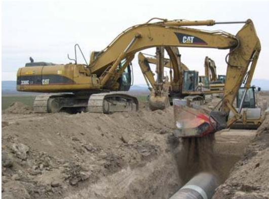
But the machine most commonly found on on-shore cross-country Pipeline projects is by far the tracked Excavator. These machines have the primary task of digging the trench, in the fastest and most economical way. With the advent of hydraulics in the late sixties, Excavators have further extended their range of application and can now perform economically in the hardest applications, while providing the reliability that Contractors seek even in the most remote locations, all over the world.
